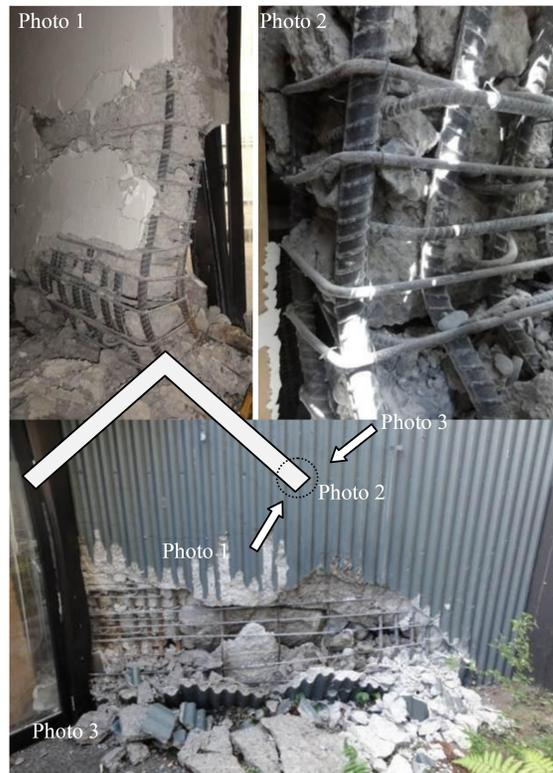
Figure 33: Seven-storey 1980s office block with significant compression failure of the V-shaped RC shear wall.
