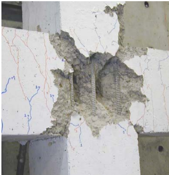
Figure 4-42: Damage Level IV, spalling of concrete at the core of the joint (Walker 2001)
